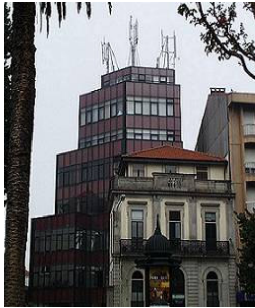
Figure 2.3 – BS antennas on a roof-top in an urban environment.
