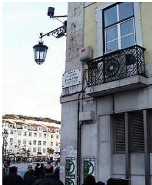
Figure 2.6 – BS antennas on a building façade in an urban environment.
