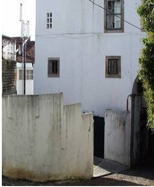
Figure 2.4 – BS antennas on a tower in an urban environment.
